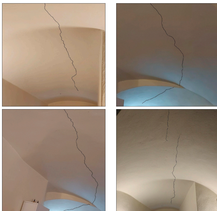
Figure 13. Damage observed on ceiling vault of the west tower at ground floor (damage ID on all four images is 13 in Figure 10a).
