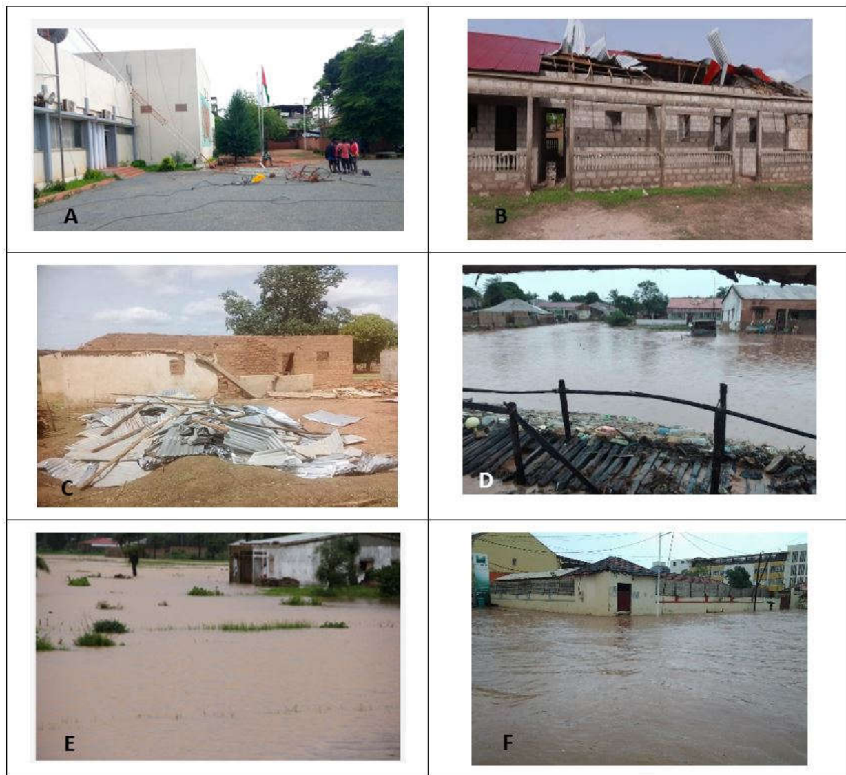
Figure 9. Flood damage in Bissau. (A)—TVGB repair work after damage caused by rain and strong winds; (B, C)—Effects of strong winds in Bissau suburbs; (D–F)—Flooded houses in the outlying neighborhoods of the city of Bissau. Sources: O Democrata GB, VISÃO, and SNPC.
