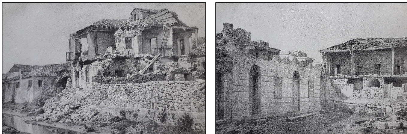
Figure 10. Typical views of structural damage caused by the 4 February 1867 earthquake to houses with load-bearing masonry walls in the town of Lixouri, located in the Paliki Peninsula. The photographs were first published by Fouqué [28], in his report on the 1867 earthquake. Partial collapse of the masonry is visible (damage of grades 4 and 5 according to the EMS-98 guidelines).
