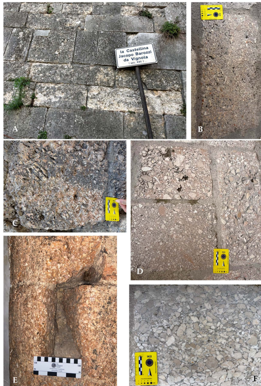
Figure 5. Breccia lithotypes from external walls (Figure 2) of Castellina (A–D): (A) Breccia ashlar of different dimensions; note the grey patina of alteration. Basement of towers with scarpa walls. (B) Polygenic breccia with red matrix. (C) Monogenic breccia with red matrix. (D) Three types of polygenic breccias with a red matrix and heterometric clasts; in (B–D), the surface of ashlar are free of grey patina, removed during the recent restoration. (E) Column of old Podestà Palace (1300 A.D.) worked in polygenic breccia with red matrix. (F) Detail of the internal staircase of the Castellina, composed of a particular lithotype with clasts belonging to the detrital levels (packstone) of the Corniola Fm.
