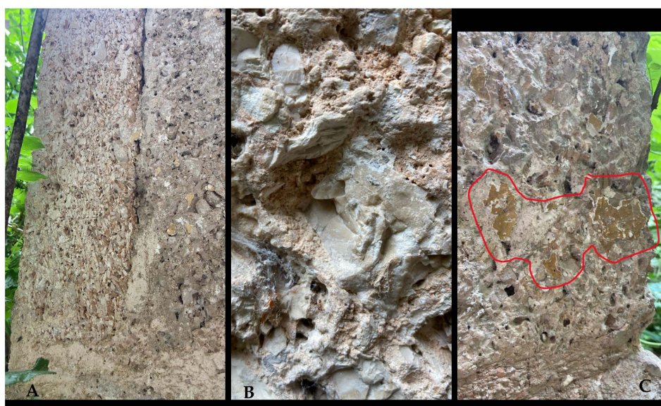
Figure 7. Breccias of cloister pilasters: (A) Two different types of breccia slabs. (B) Details of heterometric and polygenic clasts with red matrix. (C) Surface of breccia with traces of plastering (red line).
