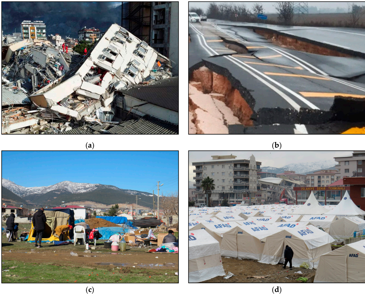
Figure 2. (a) The collapsed state hospital in İskenderun. (b) Extensive cracking and total destruction of the road due to the earthquake ground shaking resulting in permanent traffic disruption. (c) Emergency shelter set up by AFAD in İslahiye city. (d) A large part of the affected population in Turkey and Syria face adverse conditions formed by the devastating 6 February earthquakes. Lack of fresh water and emergency supplies are favorable for the emergence of infectious diseases. Photos taken during post-event field survey conducted in the field by E. Lekkas and S. Mavroulis from 7 to 11 February 2023.
