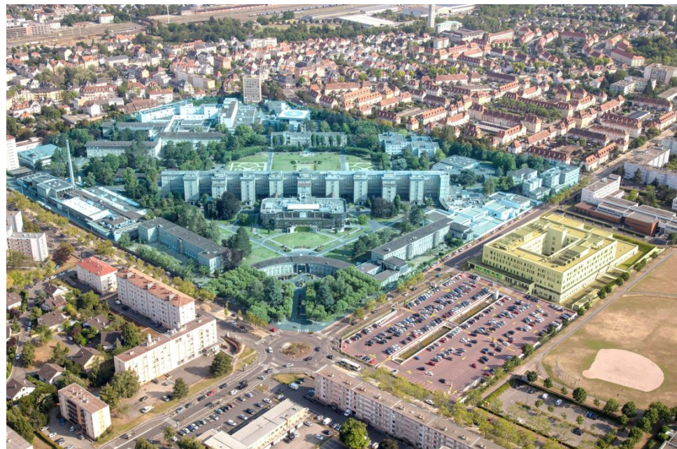
Figure 1. An aerial view of Hôpitaux Civils de Colmar with its two main geographical zones: a historic hospital (H in blue) at the center with buildings commonly built during the 20th century and having natural ventilation except in toilets with exhaust fans (558 beds, 53% are single rooms, and ACH of <1 ); and a modern hospital (M in yellow) with a square building to the right of the image that was opened in 2018 (141 short-stay beds, 91% are single rooms, with MV and ACH of >2 ).
