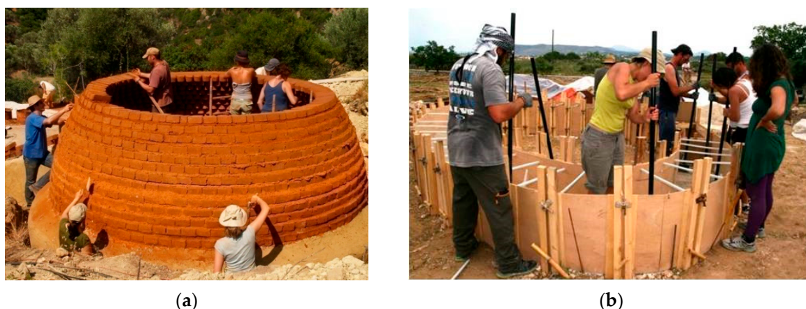
Figure 53. Piliko team: (a) Adobe construction; (b) Experimental constructions based on rammed earth technique during workshops (photos from Piliko archive).
