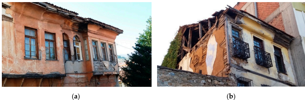
Figure 9. Veroia: (a) “Bagdati” used in sachnisi and exterior walls; (b) Sides “Bagdati” exterior walls (photos by A. Mousourakis).
