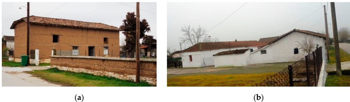
Figure 20. Thessalian plain: (a) Adobe house with wooden reinforcements; (b) Adobe rural complex (photos by A. Mousourakis).
