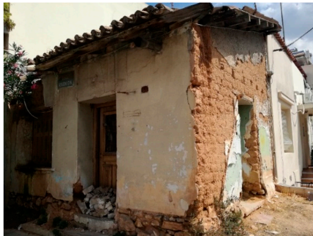
Figure 45. Nea Ionia, Athens, Kydonion, and Rodou Street, a half of the building. The second room was demolished. These are the signs of the positions from the timber framed ceiling (photo by E. Frangedaki).
