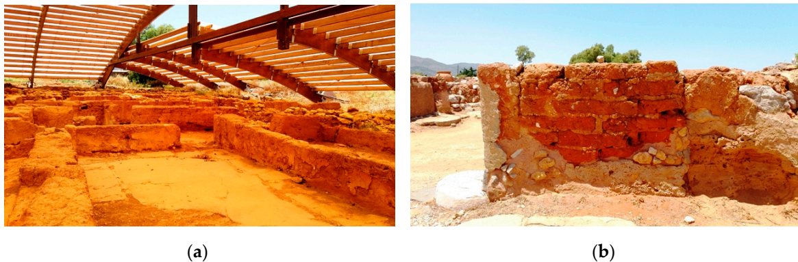
Figure 4. Archaeological site of Malia: (a) building foundations; (b) Wall made of adobe bricks coated with earth mortar (photos by A. Mousourakis).
