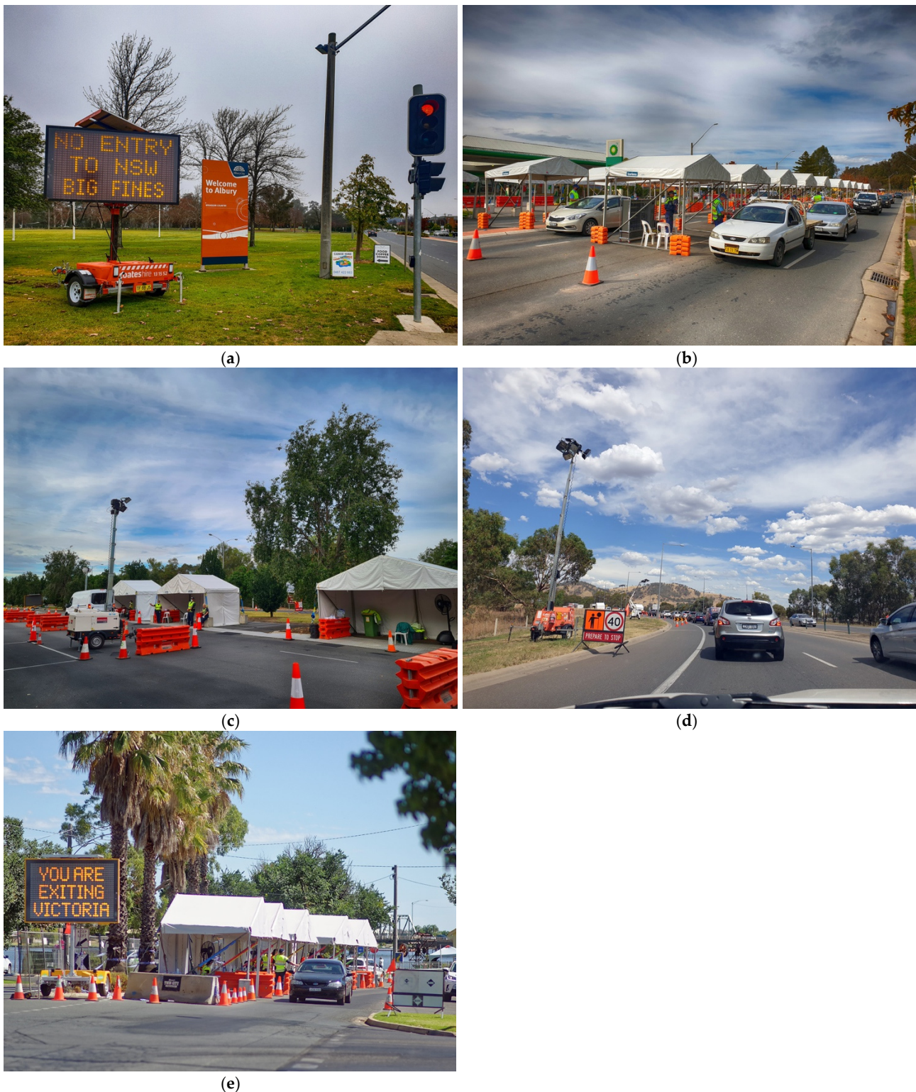
Figure 15. Temporary infrastructure for border controls between New South Wales and Victoria (Australia): (a) Trailer-mounted variable message signboards; (b) Open-sided marquees; (c) Traffic control barriers and enclosed marquees; (d) Trailer-mounted lights; (e) Open-sided marquees and trailer-mounted variable message signboards. Restrictions for Victorian residents: (a) Total border closure, 7 July 2020; (b) Travel permit checks, 9 September 2020 (both Wodonga Place, Albury, NSW). Restrictions for New South Wales residents: (c) Travel permit checks on the Lincoln Causeway, 4 January 2021; (d) Travel permit checks at the B410, 13 January 2021 (both Wodonga, Victoria); (e) Travel permit checks at Yarrowonga, 12 January 2021 ((e) Source: Wikimedia Commons).
