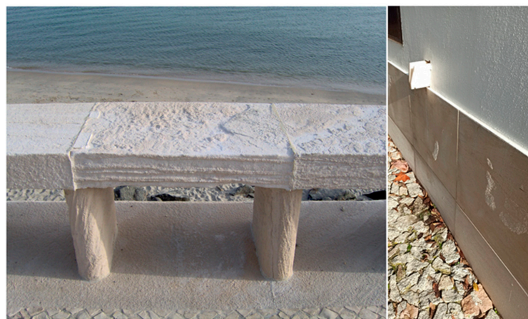
Figure 2. Examples of limestone elements subjected to natural salt weathering in a coastal area (photo credits: Joaquim Simão and Carla Lisci).
