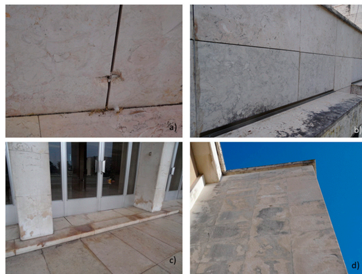
Figure 1. Examples of natural stone facade reactions to environmental conditions: (a) anchor rupture leading to strength loss; (b) biocolonization showing a relevant colour change; (c) white stains from saline efflorescence; (d) dark stains from water absorption, which might lead to slab detachment (photo credits: Vera Pires).
