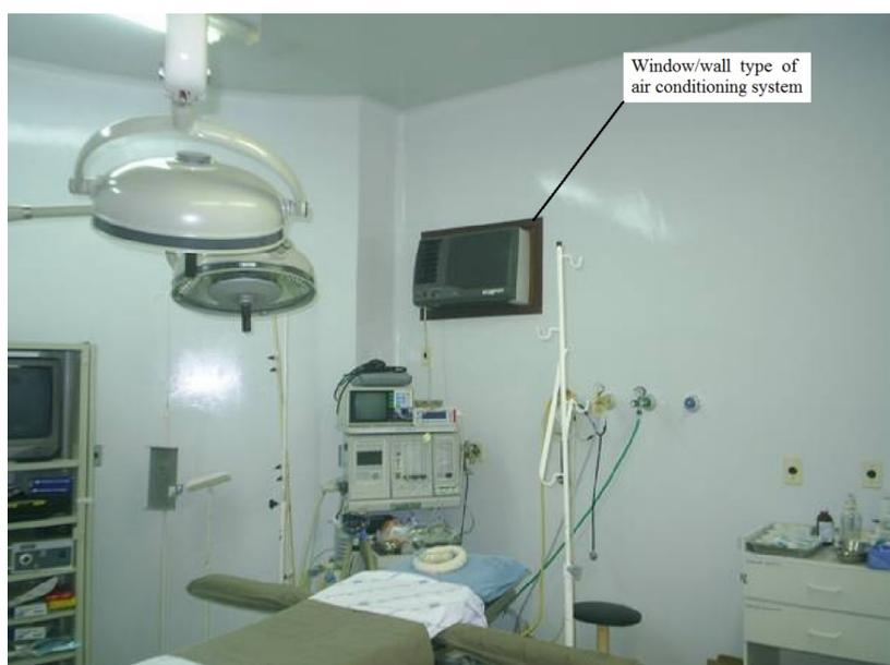
**Figure 1.** Surgical room and window/wall air conditioning system in which the  $CO_2$  and particle concentrations were measured.
