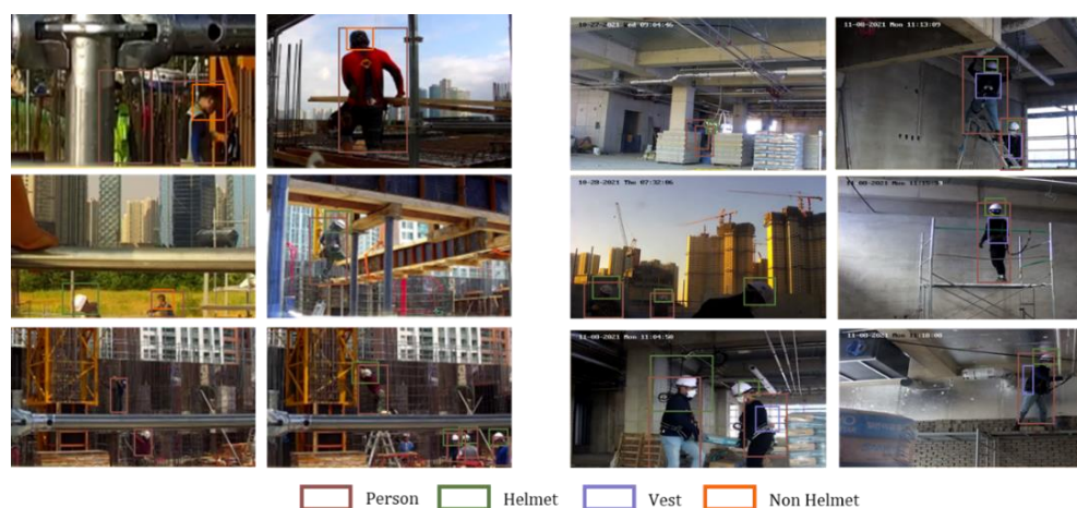
Figure 16. Analysis result of image sample using YOLO v2.
