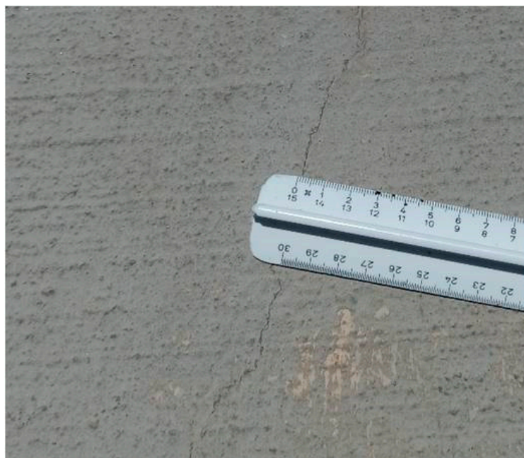
Figure 6. Example of a shrinkage crack.
