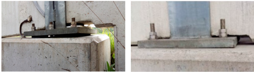
Figure 3. Different designs and qualities of fixing the steel posts of NB to the concrete edge beam.
