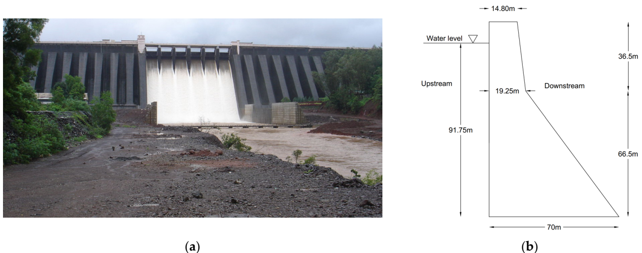
Figure 6. Koyna Dam (a) downstream view [41], (b) cross-section [42].
