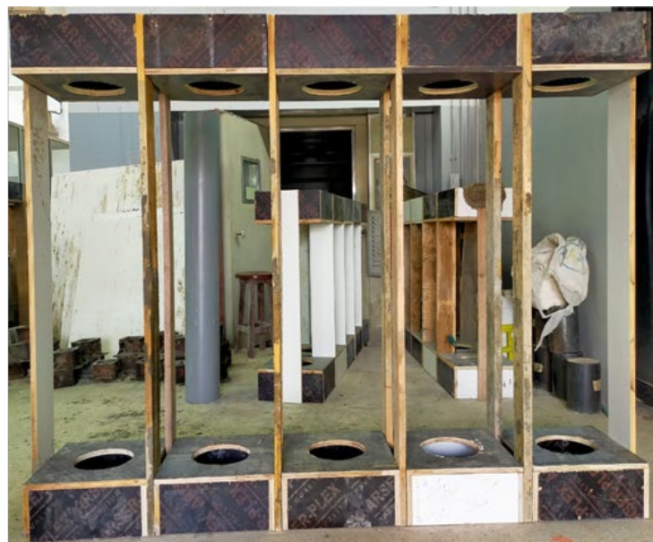
(b) Preparing formwork and placing the PVC
