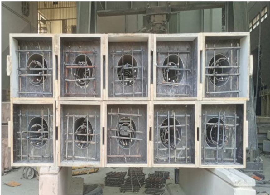
(c) Placing the cage of reinforcement in the formwork
