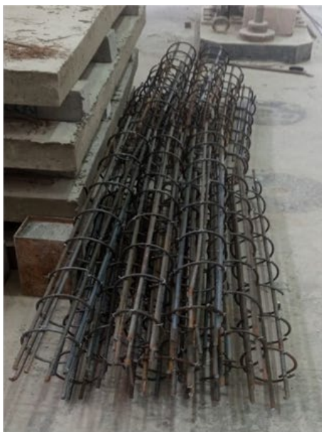
(a) Preparing cage of reinforcement
