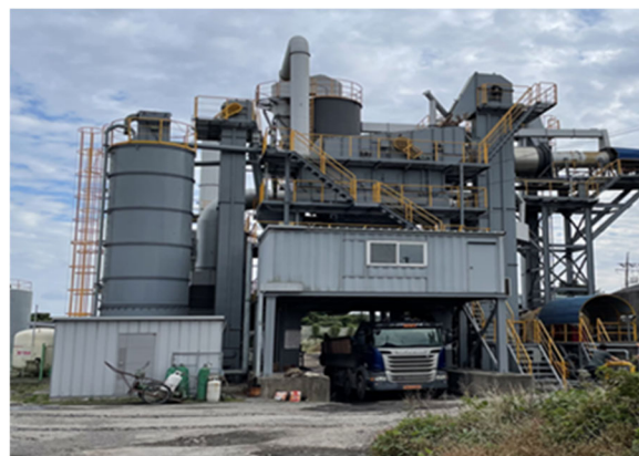
Figure 5. Seoil asphalt plant to produce Zero-M mixtures in Seogwipo City, Korea.
