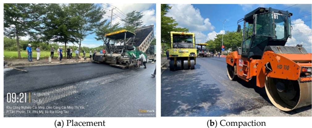
Figure 13. (a) Placement and (b) Compaction of Zero-M PCMA Mixtures.
