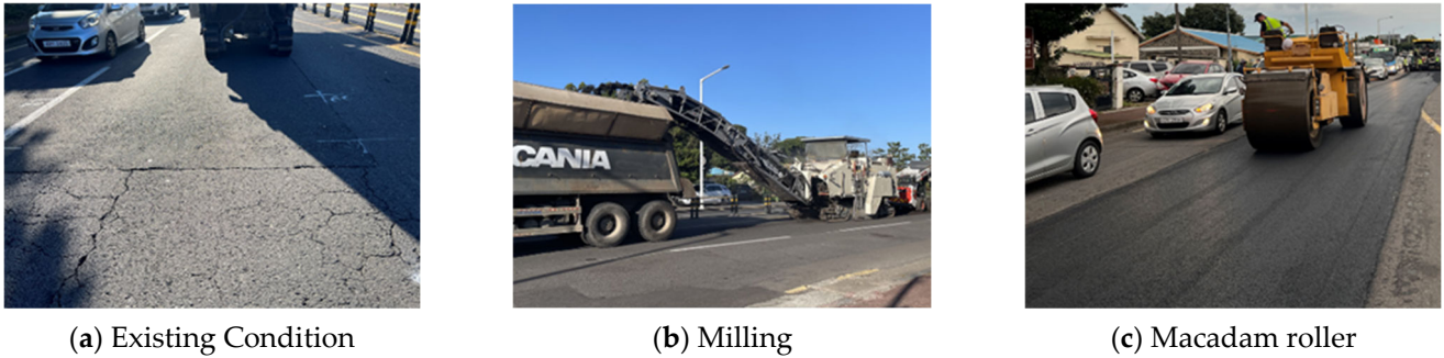
Figure 6. Construction of 150 m-long “Zero-M” PCMA test section in Seogwipo City, Korea.
