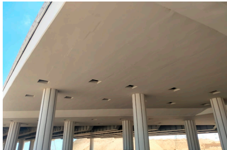
Figure 14. Coating with acrylic polyurethane paint.
