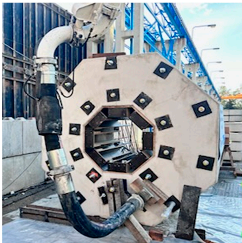
Figure 6. Pumping concrete into the lining.
