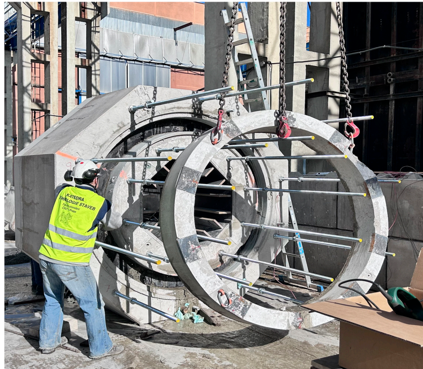
Figure 10. Removal of concrete plunger to check the final condition of the concrete.
