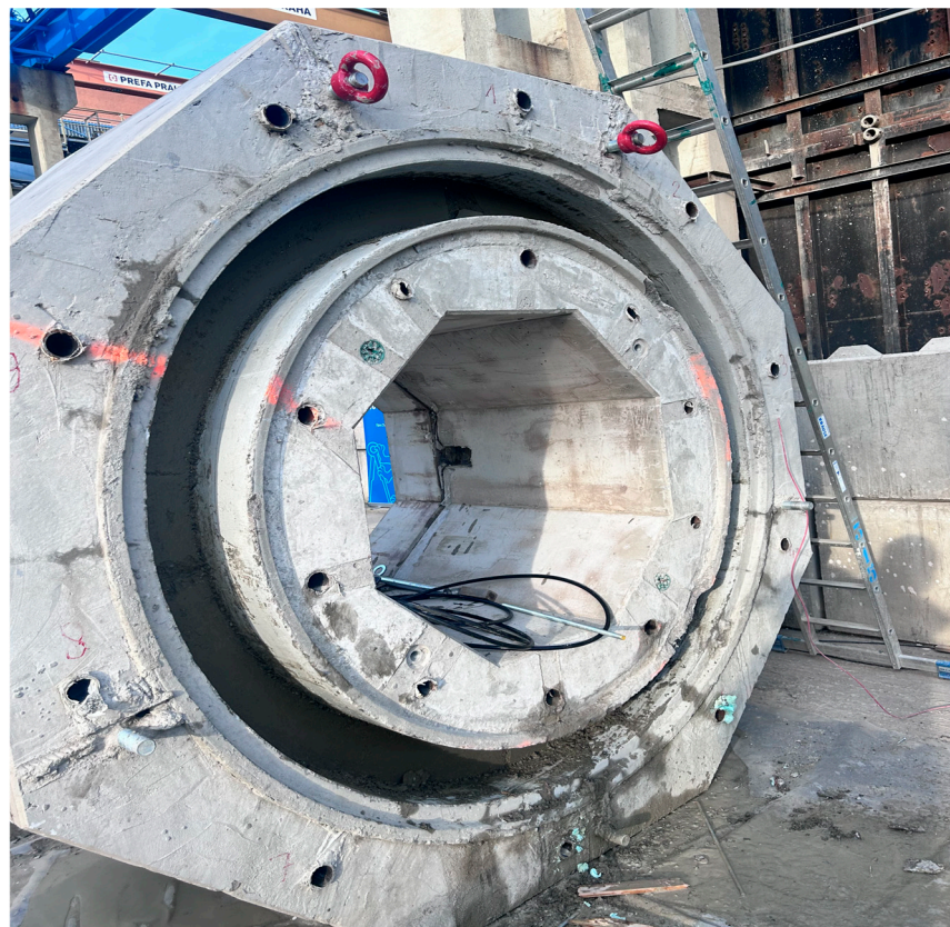
Figure 11. The final state of the concrete after 90 min of pumping.
