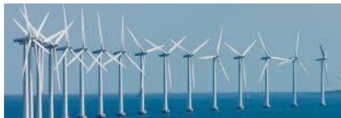
Figure 12. Wind turbine farm [82].
