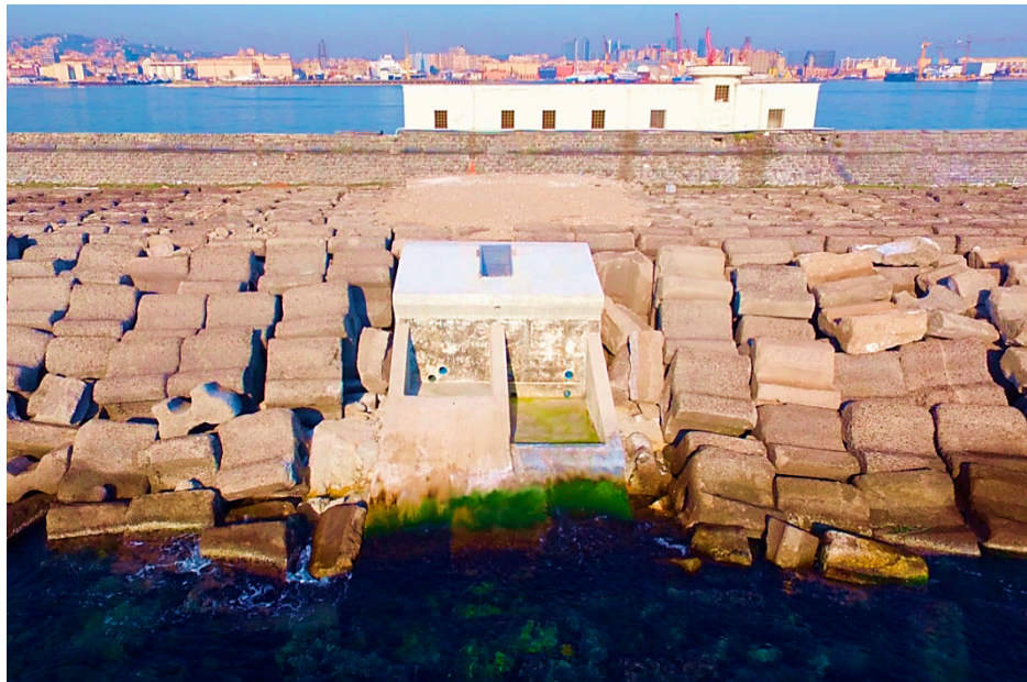
Figure 13. The OBREC prototype installed in the San Vincenzo breakwater, port of Naples.
