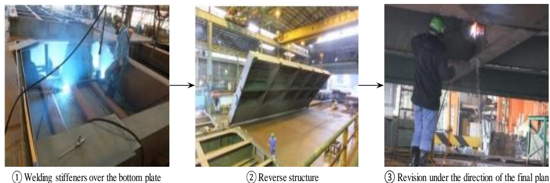
Figure 16. Welding work process of a hatch cover.
