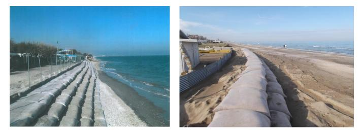
**Figure 1.** Application of "Stopwave" as coastal revetments: Grottammare, Italy (**left panel**) and Senigallia, Italy (**right panel**).
