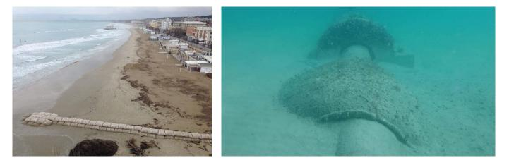
**Figure 2.** Application of "Stopwave" as temporary groin in Senigallia, Italy (**left panel**) or as pipeline protection (**right panel**).
