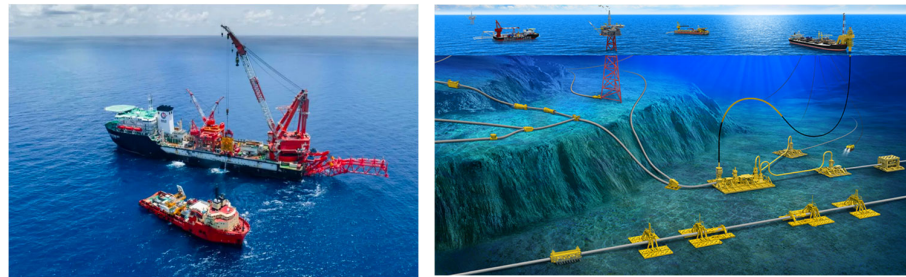
Figure 1. Laying of subsea pipelines (left) and a crisscrossing subsea pipeline network (right).
