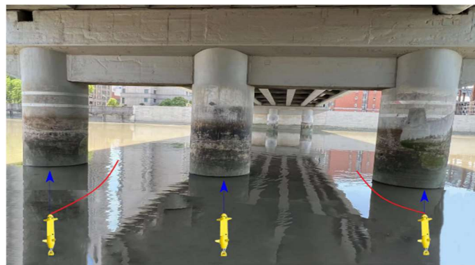
Figure 1. Multi-AUV system performs the bridge detection.
