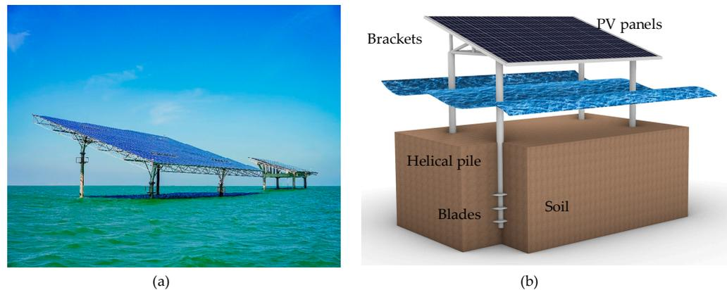
**Figure 1.** Fixed offshore PV: (a) First fixed offshore PV in Shandong Province, China; (b) Helical piles for fixed offshore PV foundation.
