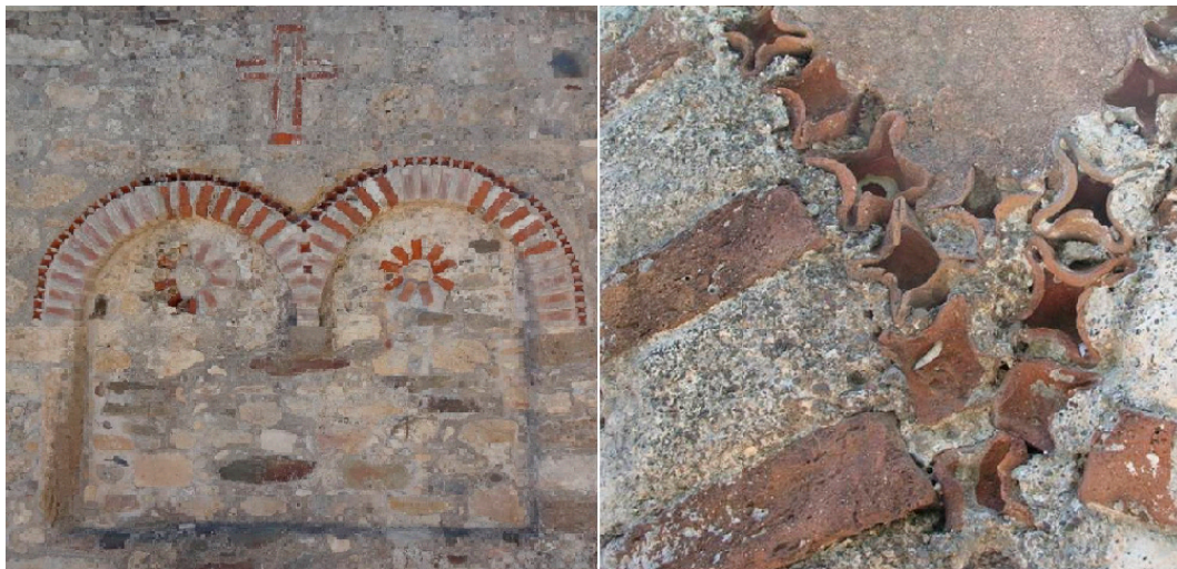
Figure 19. Detail of brickwork and rosettes on the facades of the Kato Episkopi Siteias church (bath-house). (Photo: A. Tantsis).
