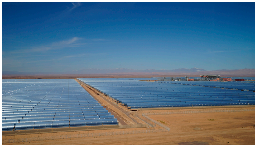
Figure 2. Noor Ouarzazate Solar Project complex (Photo: Sarah Ryser 2018).
