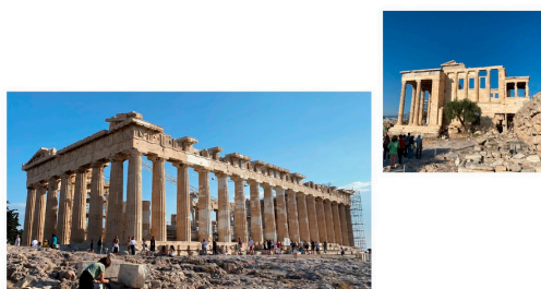
Figure A1. Photographs used to represent Classical architecture in questionnaires for Athens.
