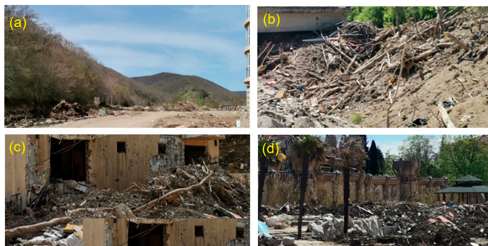
Figure 10. Flood debris and waste, over half a year after the disaster: (a) the flat part at the transition between the mountainous and built-up areas; (b) the place where the river flow enters the underground passage; (c) flood debris downstream; (d) destroyed attractions.
