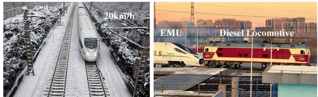
Figure 2. A typical situation of severe icing on the contact network in Hubei during the 2024 Spring Festival travel rush.
