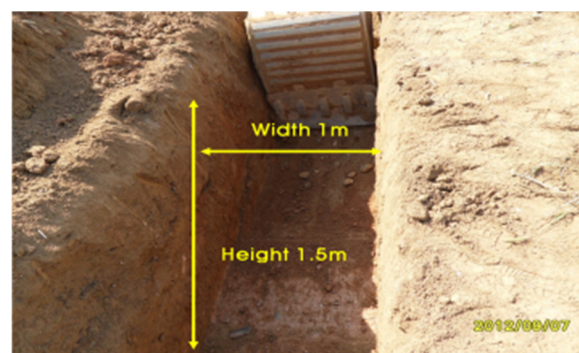
Figure 11. Trench excavation for the plastic foundation.
