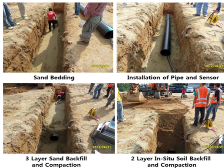
Figure 12. Field construction process.
