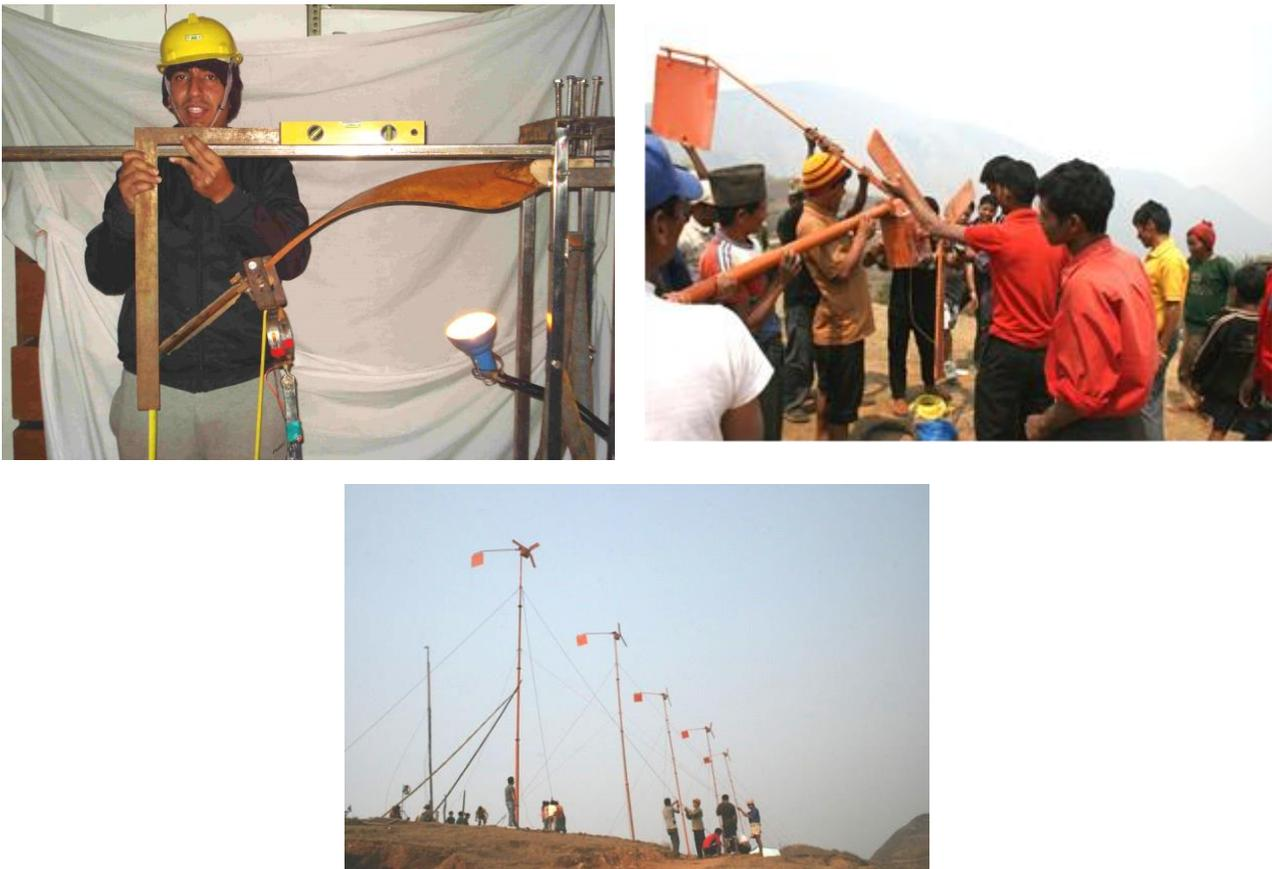
**Figure 10.** Locally produced wooden wind turbine in Nepal: testing and installation in Dhulikhel region. The figures are reprinted from [147] with kind permission of Elsevier.
