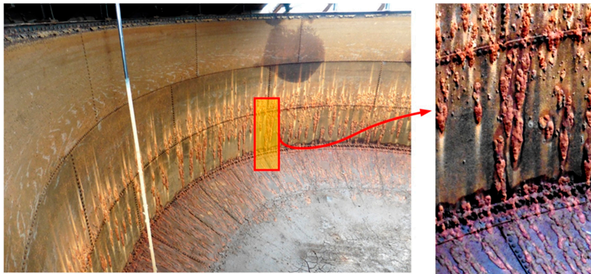
Figure 2. View of a fragment of the interior of the steel tank in the tower.
