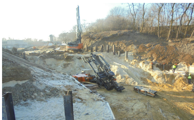
Figure 5. Passage of the communication corridor through the anthropogenic embankments: construction of the soldier pile wall. Clearly visible uncovered substrate layers of different colors.
