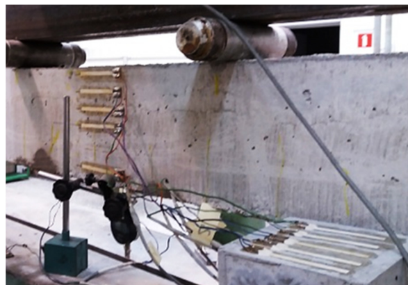
Figure 3. Strain gauge placement.
