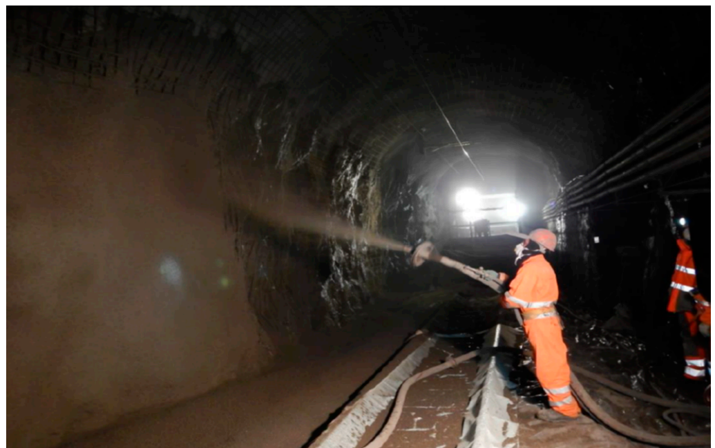
Figure 4. Shotcrete spraying around a tunnel sidewall.
