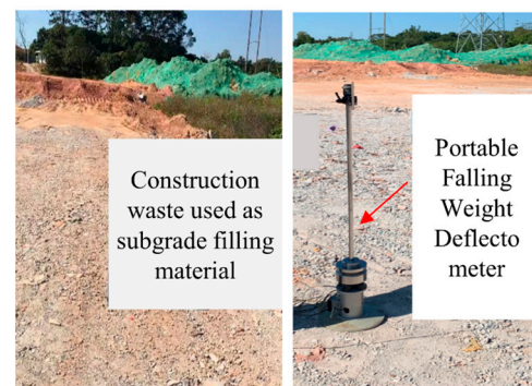
Figure 6. Recycled construction-solid-waste aggregate used for subgrade filling.
