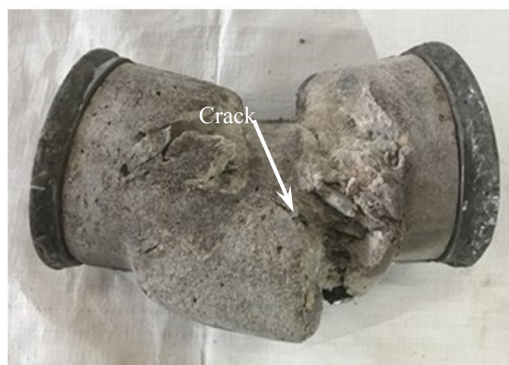
(a) Overall failure of concrete
