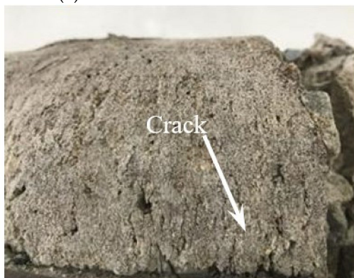
(c) Concrete tensile cracking
