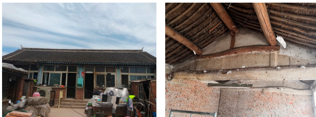
Figure 1. Timber-framed masonry structure.
