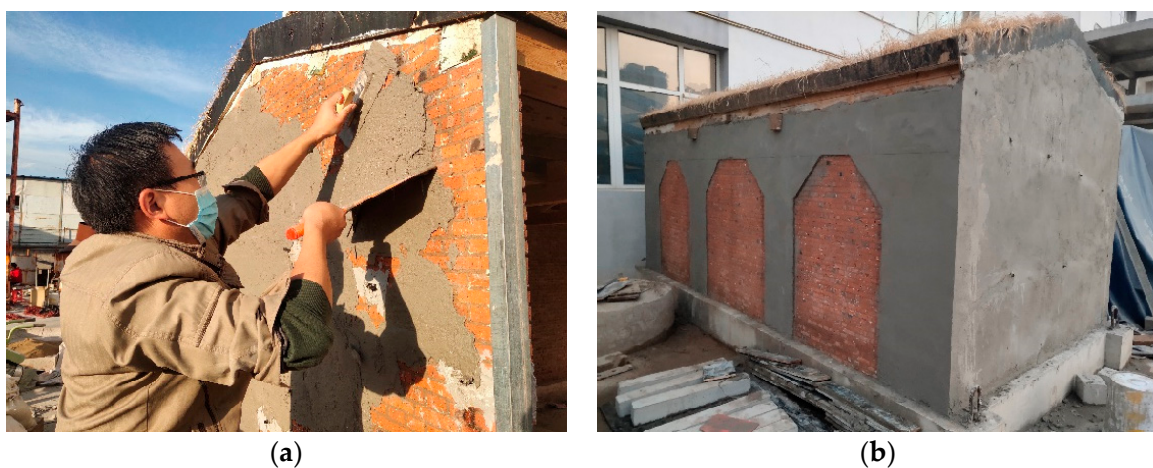
Figure 5. Model reinforcement process and effect: (a) Model reinforcement process; (b) model reinforcement effect.
