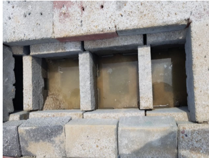
Figure 16. Rainwater storage condition of the storage block.
