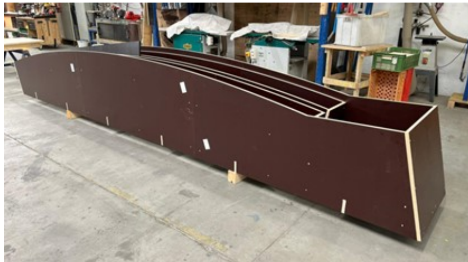
Figure 6. CNC-milled formwork assembled from smooth plywood panels for the casting of UHPFRC arch segments.
