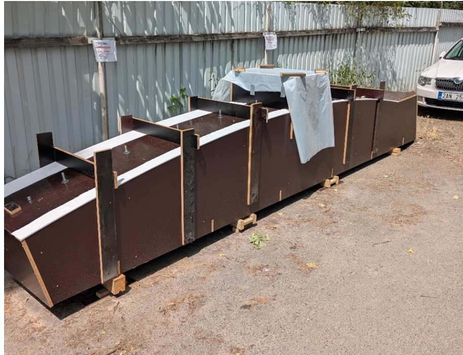
Figure 7. Casting of UHPFRC into the assembled formwork; filling was performed in stages and monitored through inspection and venting openings.
