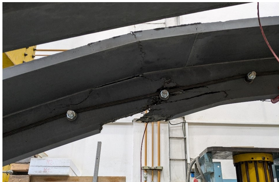
Figure 14. Experimental detail of second crack.
