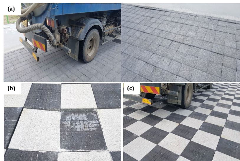
Figure 16. Pavement stability after field vehicle loading: (a) Zone A, (b) Zone B, and (c) Zone C.
