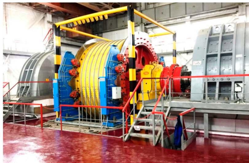
Figure 1. External view of the shaft hoisting plant.
