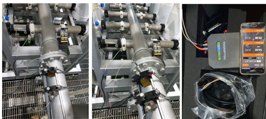
(a) Sensor and transducer (clamp-on type)
