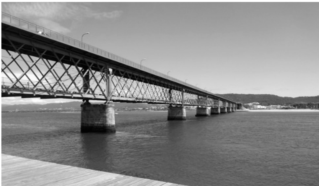
Figure 1. A view on the Eiffel Bridge.
