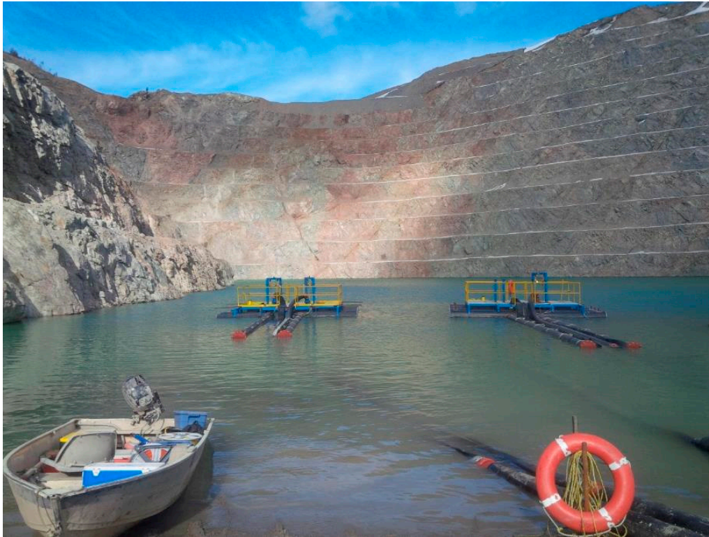
Figure 8. Springer Pit Lake and dewatering infrastructure at Mount Polley Mine, BC, Canada.
