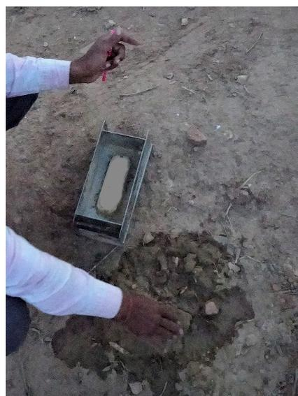
**Figure 6.** Silty clay surface sediments are first wetted, then pressed into brick-shaped molds in the area adjacent to the kiln. Photograph by: P. Chirico.
