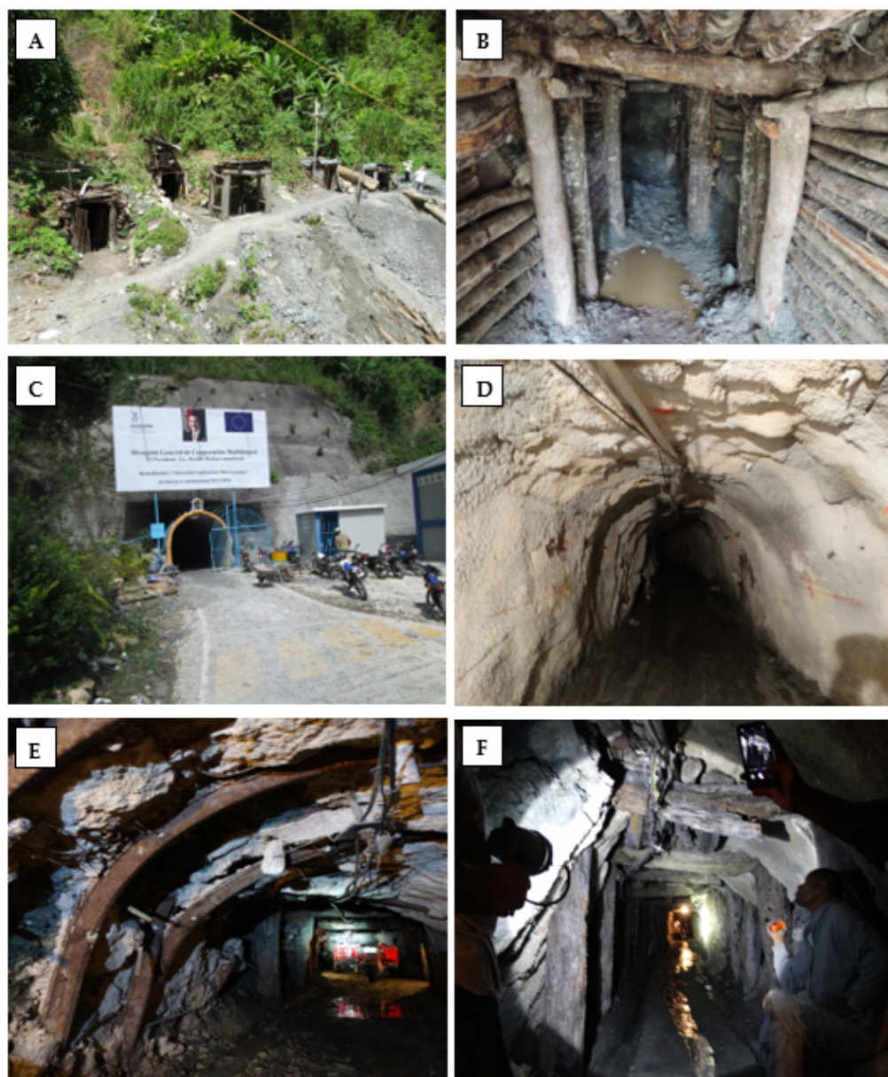
Figure 3. Mining of larimar in basaltic rocks at the Las Filipinas mine. (A,B) Shallow excavations in the slope of the hill with a primitive timber lining (as of 2013); (C,D) tunnel with steel and timber support and concrete rendering (as of 2016); (E,F) tunnel as of 2020; Photographs were taken by L. Natkaniec-Nowak and K. Broda.
