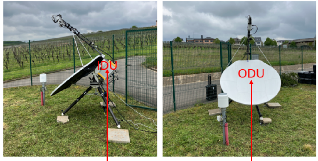
Figure 6. Fixed Edge Node installation at the vineyards in Remich, Luxembourg: Outdoor Unit (ODU) + Indoor Unit (IDU).
