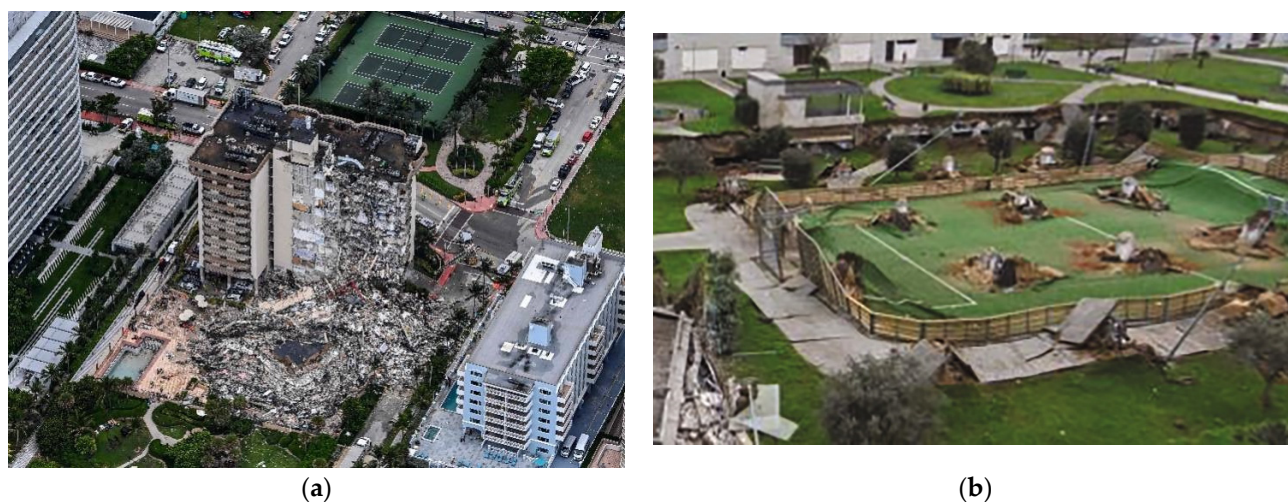
Figure 1. Collapsed of (a) condominium building [1] and (b) a parking garage on a playground [2].
